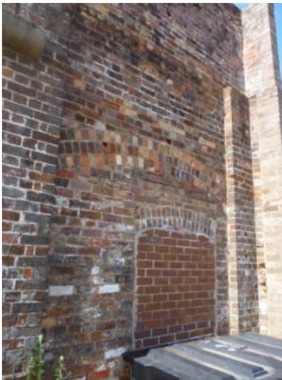
Figure 11: Southern c1865 façade views of the subject site, showing the deteriorated and poor condition of the brickwork, which was once an internal wall for the remainder of the original factory, which was demolished in the 1970s.
